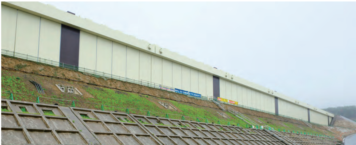
Construction work to raise the seawall (Onagawa Nuclear Power Station)
