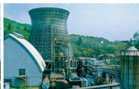
Matsukawa Geothermal Power Station (Hachimantai City, Iwate Prefecture)
