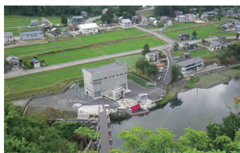
The No.2 Yabukami Power Station (Uonuma City, Niigata Prefecture)
