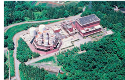
Yanaizu-Nishiyama Geothermal Power Station (Yanaizu Town, Fukushima Prefecture)
