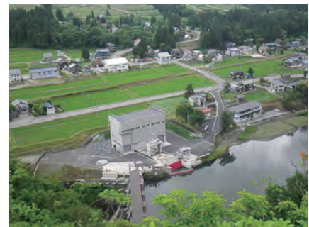
The No.2 Yabukami Power Station (Uonuma City, Niigata Prefecture)
