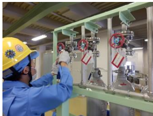
Training on replacing nitrogen gas cylinders for use in the bulb operation to prevent excessive pressure in the pressure vessels (Onagawa)
