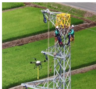
A scene from power line extension works using drones (August 2021)
