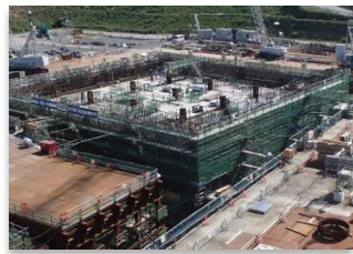
Emergency response facility (Onagawa: Building body construction)
