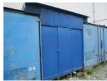
N3_鋼製物置(3)
