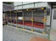
N5_仮設足場(1)
