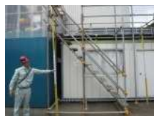
N3_仮設足場(1)
