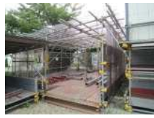
N5_仮設足場(2)
