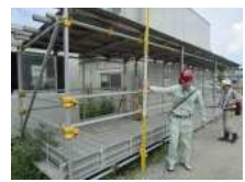
N5_仮設足場(5)
