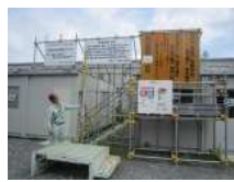
N5_仮設足場(4)
