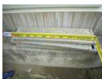
CN3_仮設足場板(2)
