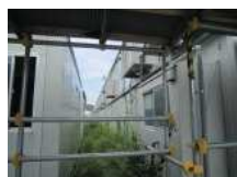
N5_仮設足場(6)
