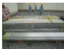
CN3_仮設足場板(1)
