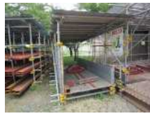
N5_仮設足場(3)
