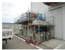
N3_仮設足場(3)
