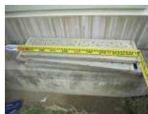
CN3_仮設足場板(2)
