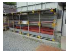
N5_仮設足場(1)
