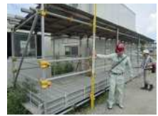
N5_仮設足場(5)
