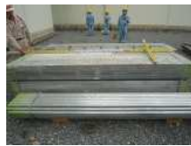
CN3_仮設足場板(1)
