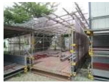
N5_仮設足場(2)
