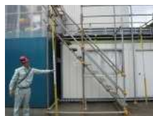
N3_仮設足場(1)
