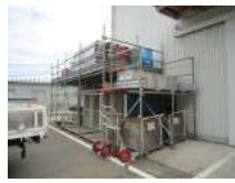
N3_仮設足場(3)
