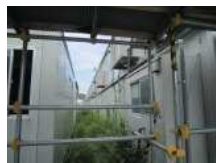
N5_仮設足場(6)
