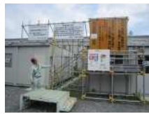
N5_仮設足場(4)
