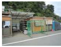
N3_仮設足場(2)
