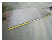
N1_敷き鉄板(1)
